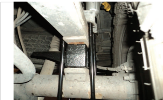
Raise axle and secure block with new u-bolts and hardware.
