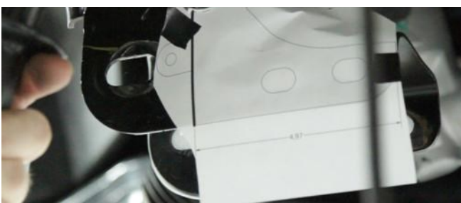
INSTALL THE TEMPLATES AND CUT
