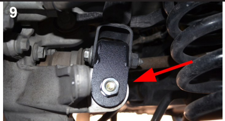
Install lower shock extension to shock and knuckle.
