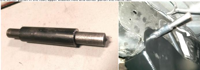
17. Remove the sleeve and punch and use a pilot bit to drill the center-punched hole. Then, use the provided 3/4" hole saw to drill the frame to match the rear bracket hole.
