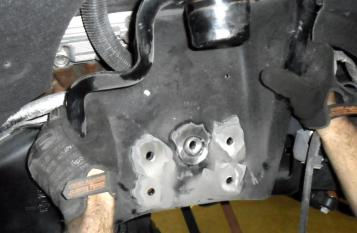
7. Install upper Coil Bucket with supplied ½" hardware and torque hardware to 85 lb/ft Torque the bottom bolts first to ensure the bracket is tight to the frame.
