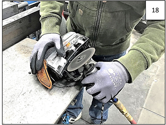
Using a cutoff wheel or saw, cut 4 plastic tabs on light housing as shown.
