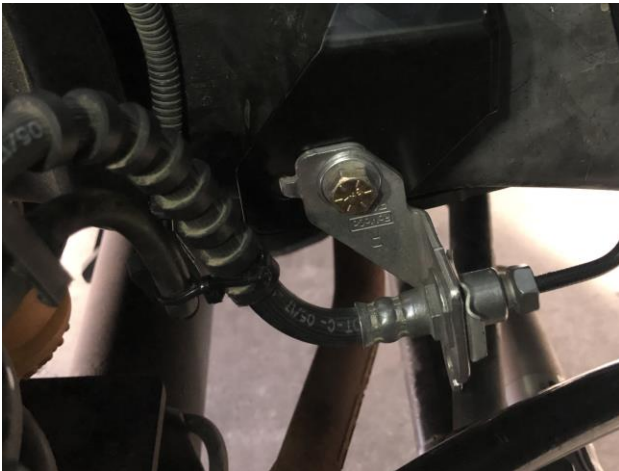
Figure 5: Driver Side ABS Line Installed
